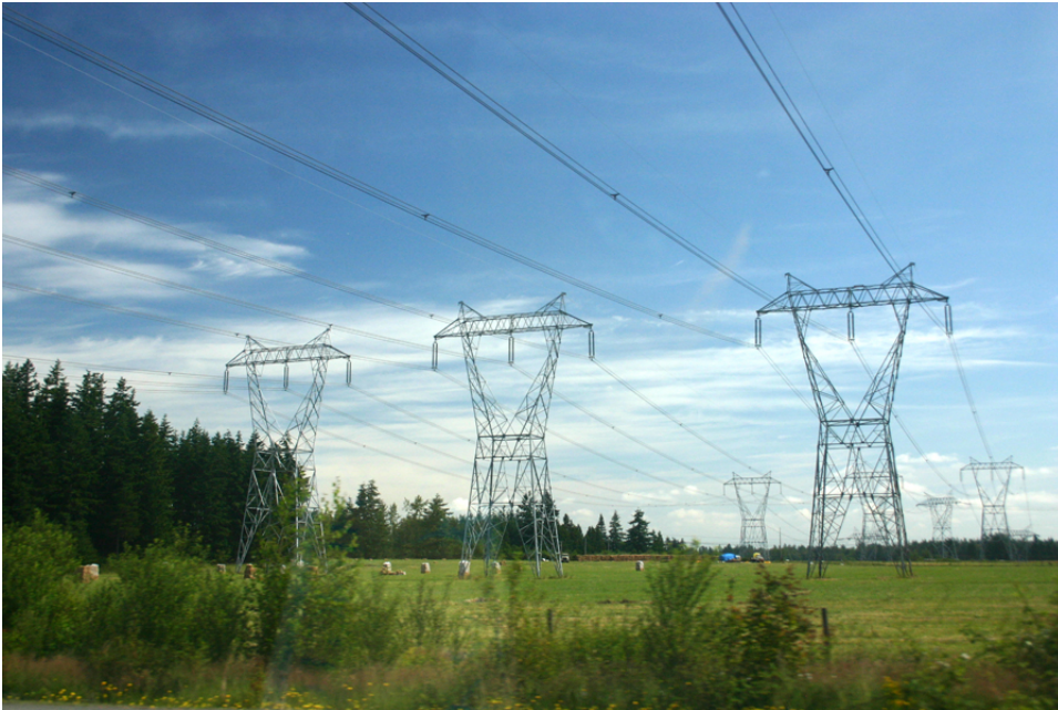
Three-phase power distribution lines. 1
